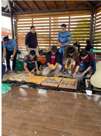
Figura 2: Practical scale quinchá workshop (Source: authors, 2024)
