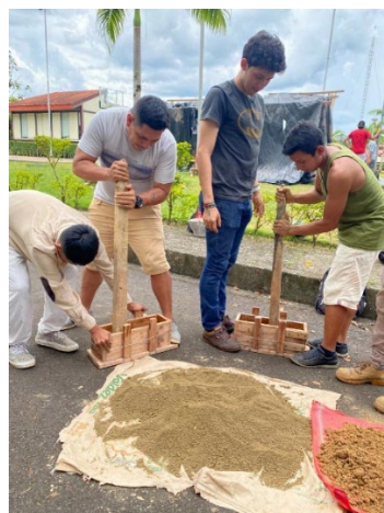
Figure 1: Practical workshop of a scale mud wall. (Source: authors, 2024)
