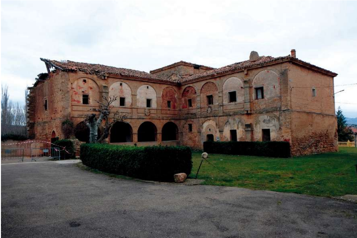
Figure 1: South and West façades of the building. Original condition 2022. (Source: Paula Montoya, Architect)
