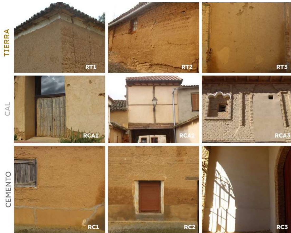
Figure 1.- Different examples of coatings on raw earth walls, Tierra de Campos region (Spain)
