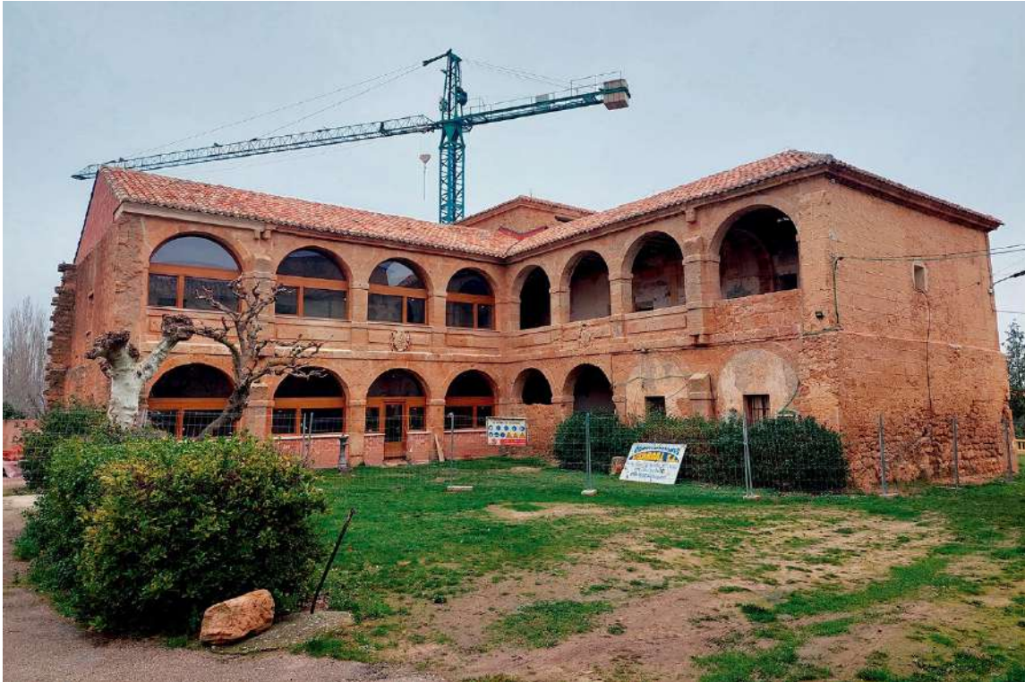
Figure 2: South and West façades of the building. Onsite works in January of 2024. (Source: Paula Montoya, Architect)
